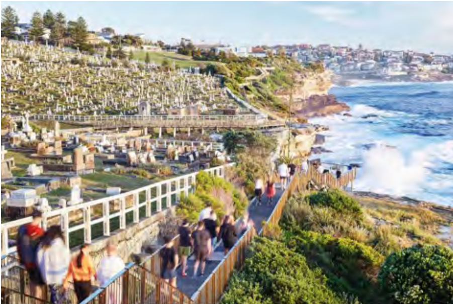
Extension of the Bondi-Bronte Promenade. Source: ASPECT Studios, https://landezine.com/bondi-to-bronte-coastal-walk-extension-by-aspect-studios/
